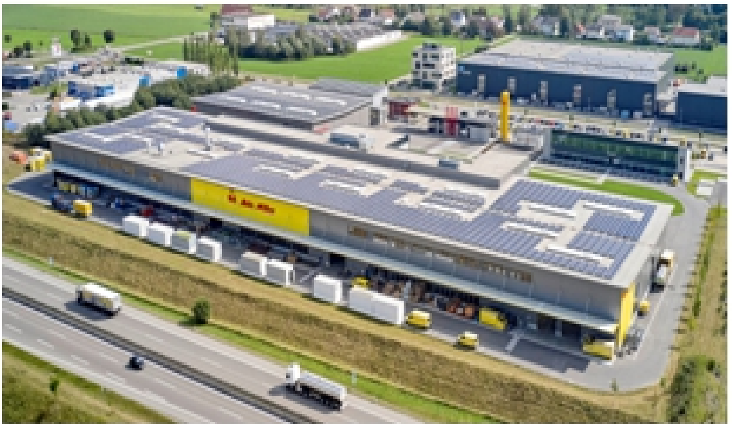
Climate-neutral factory with photovoltaic systems (Source: Alois Müller GmbH)
